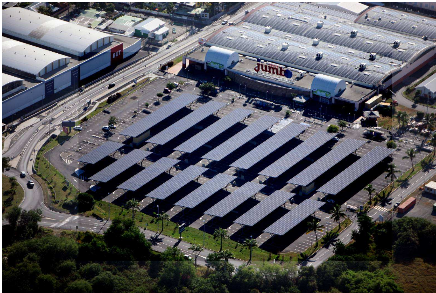
Saint-Paul (La Réunion) – 2,500KWp - Operational since August 2010
