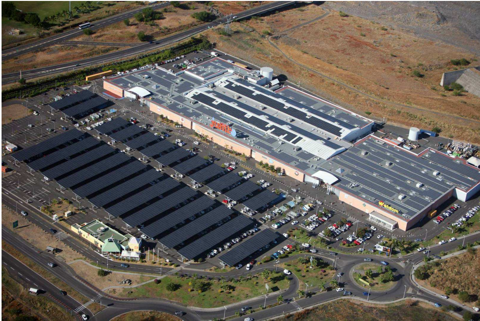
Le Port (La Réunion) – 3,900KWp – Operational since September 2010
